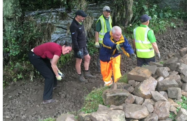
Volunteers clear debris from Langthwaite bridleway
